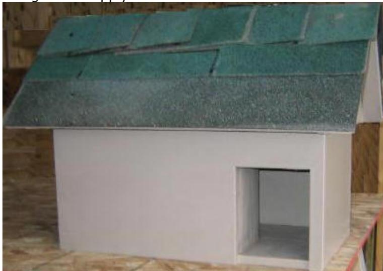
**Step 5, Finish the House-** Apply edging material, fill all holes with wood plugs and/or filler, sand, and apply stain/poly or paint; seal the floor against moisture. Once the poly has cured, apply carpeting to the floor and a flap door. Find your cat and stick it in there.
